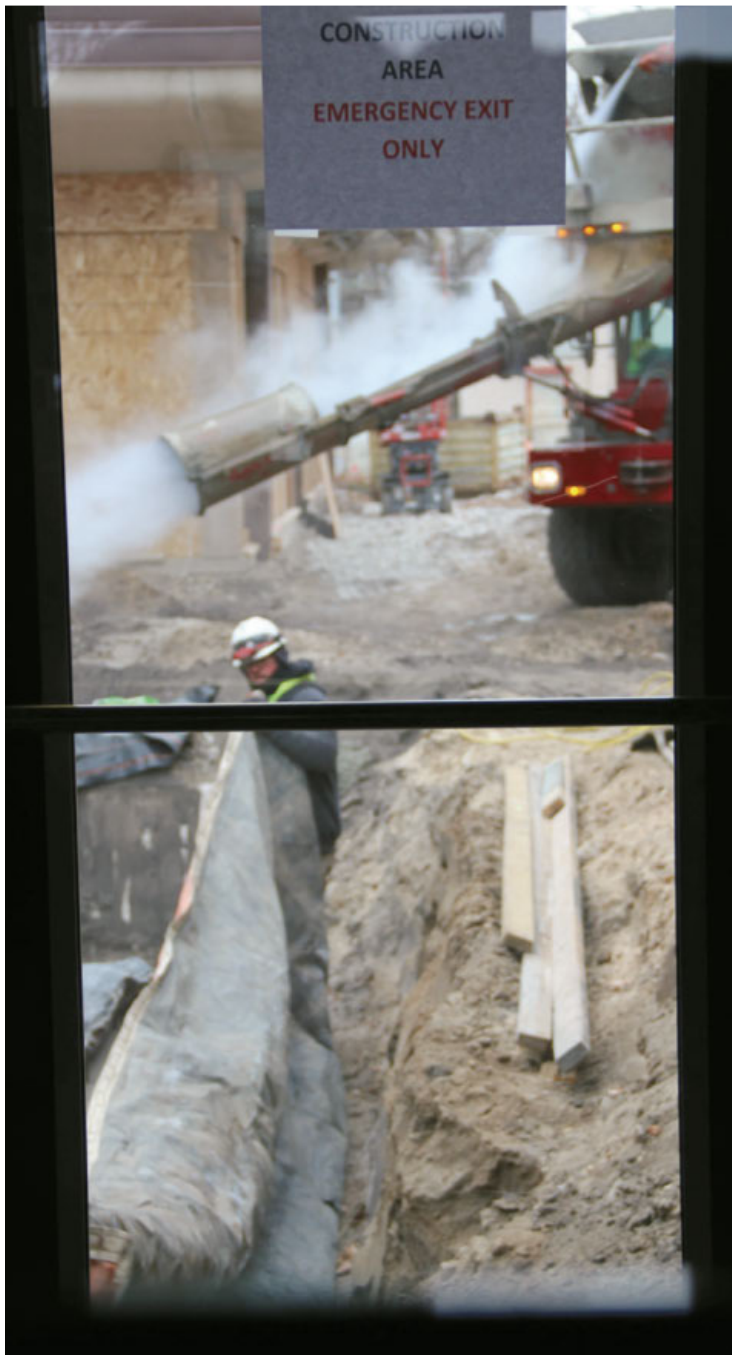
The cement footings have been poured for the new gathering space between the church and the parish center.
