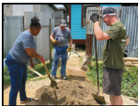
Mixing concrete for front porch (Desiree Burgess, Mark Enderlin, Don Kremer)
