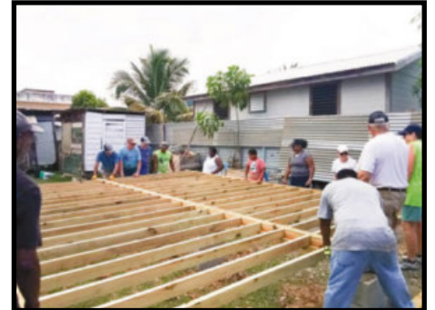
Positioning floor frame on foundation
