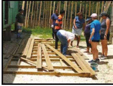
Assembling a Wall at Hand in Hand HQ
