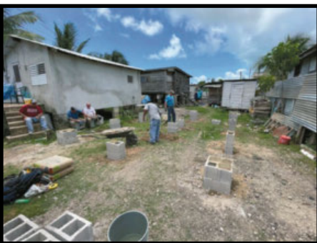
Men preparing foundation of house at Desiree's plot
