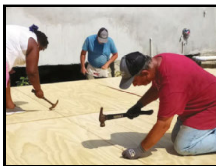
Nailing plywood floor
