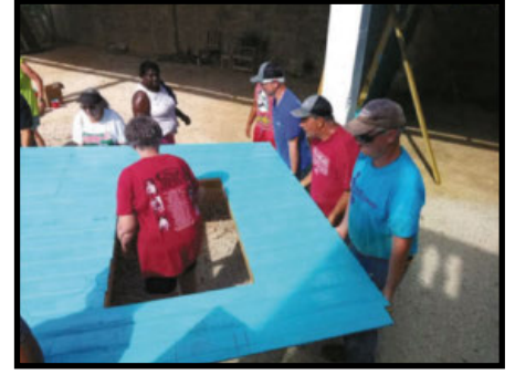
Moving painted wall to truck to move to site
