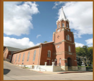
ST. MARY PARISH 400 Franklin St. Galena, IL
