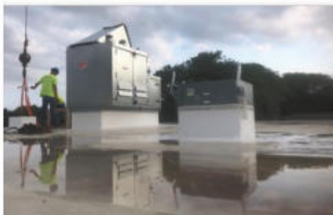
New makeup air unit set on the new curb.
