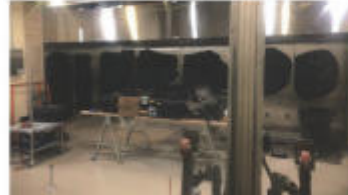
Stainless walls panels on fryer wall
