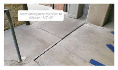
Uneven sidewalk slabs and cracks pose a trip hazard and liability. We have received an estimate from Hoffman Construction to remedy 6 areas of concrete.
