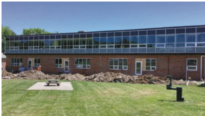
Photo of the Borromeo Academy window and door replacement work on the back side area facing the Early Childhood activity deck and play area.
