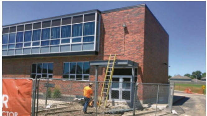
Photo of the new Borromeo Academy Early Childhood front entrance installation.
