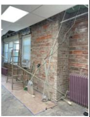
Renovation is in full swing on the school walls. The old outer walls have been torn out, metal studs have been installed, new electrical conduit has been installed and drywall is going up. The sealing and tuckpointing of the school building should start soon.
