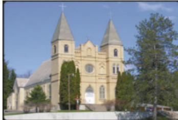
ST. STANISLAUS Sobieski, Minnesota 9406 Church Circle Little Falls, MN 56345 **Office Address**
