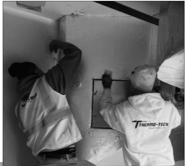
Above: Duct work from the air handler is being sealed off on the exterior wall finishing up the installation.
