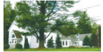
St. Paul's 771 Route 29, Rock City Falls
