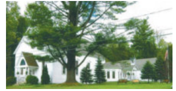
St. Paul's 771 Route 29, Rock City Falls
