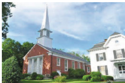
St. Anthony of Padua Church Located at 49 South Street, P.O. Box 97, Litchfield, CT 06759 860-567-5209 stanthonypadua@optonline.net
