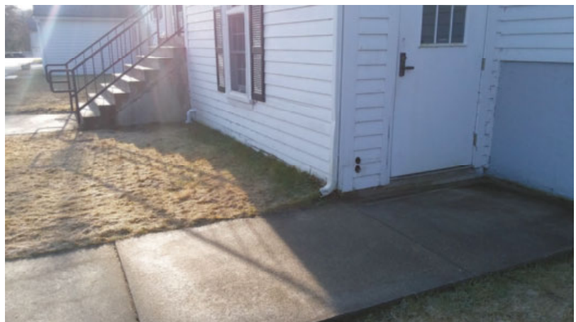
Above: Rear of church; both roof drains put into new underground pipes; larger capacity
