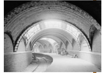
The City Hall station of the IRT Lexington Ave. Line
