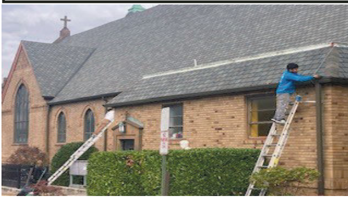
Gutters cleaning and repairs at St. Paul's
