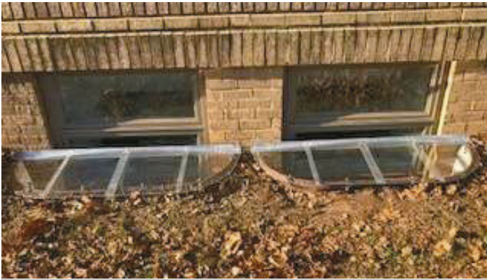
St. Paul's Church Repairs Completed
