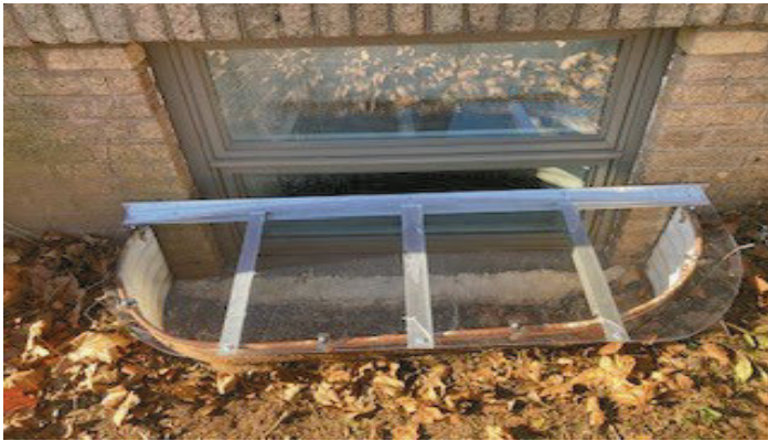
St. Paul's Church Repairs Completed
