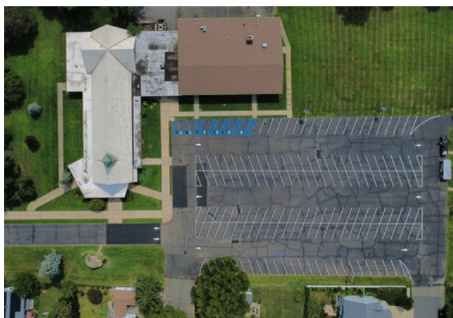
Guardian Angels Parking Lot Repair: Patching, Cracks cleaning and filling, and restriping
