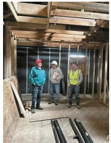
Photos of the construction of Saint André House by John Goddard.
