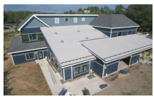
Walkways have been installed, including a pad for the emergency generator. Concrete walkways in the front of the building are nearing completion and landscaping has commenced. The parking lot has been paved with a base coat. Final coating and sealants will be applied as weather dictates. Storm drainage systems were put to the test with recent rains and successfully dealt with the deluges.
