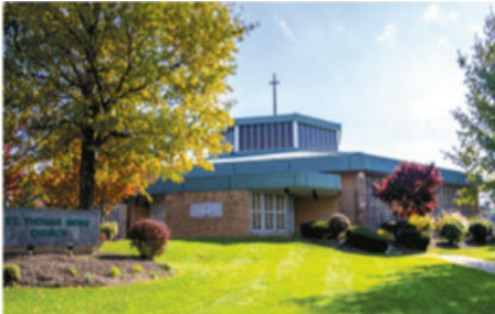
St. Thomas More Church Address: 126 Fort Couch Road Pittsburgh, PA 15241 Parish Office: 412-833-0031 Ave Maria Academy: 412-833-1412
