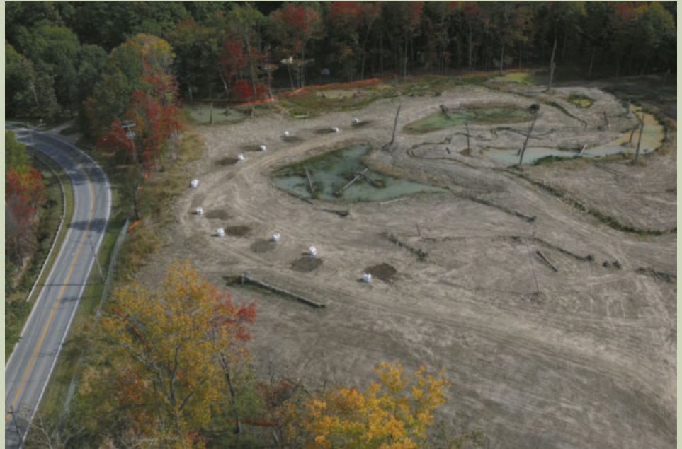
A drone shot of the former Padua soccer fields shows how the property looked when transferred to Cleveland Metroparks last December.
