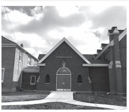
New addition and renovation at St. Mary, Our Lady of the Annunciation, Rockwood
